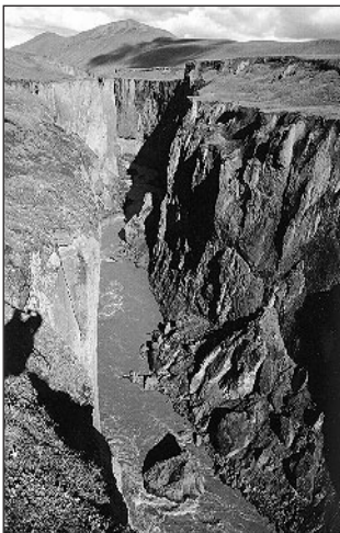
The dam is being built at the head of this canyon.
