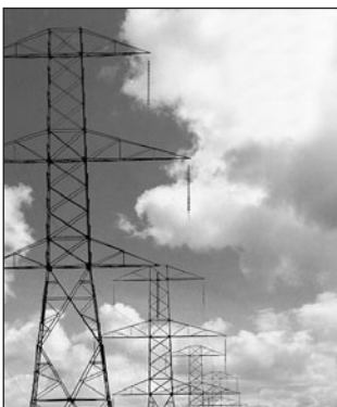
Clearly visible high voltage power lines are a problem.
