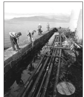
Oil tanks are surrounded by walls to protect against pollution.
