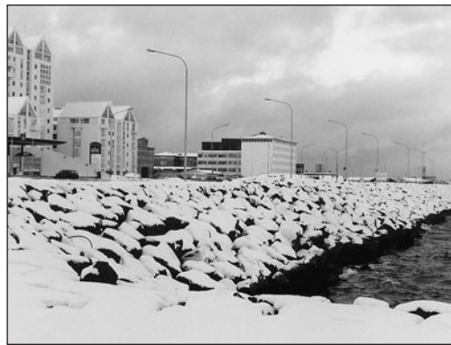
Rough breakwaters destroy the possibility of using the coast.
