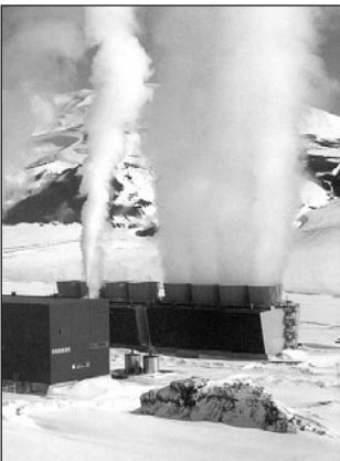
Krafla is Iceland's second largest steam power plant.
