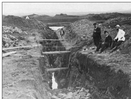
This ditch for the water pipeline from Gvenndarbrunnur was dug manually.
