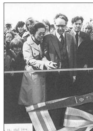
Cutting the ribbon. Ring Road opening in 1974.
