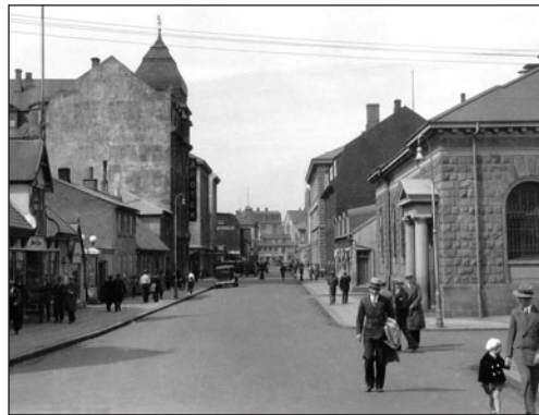
Continuous lines of houses means that fire-safety walls are visible until the street lines have been completed.
