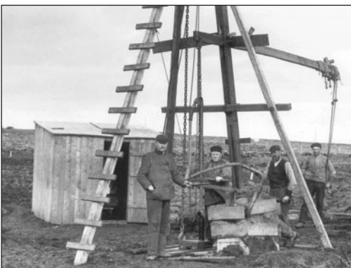
This drill was bought for drilling for cold water but later struck gold by getting geothermal water.
