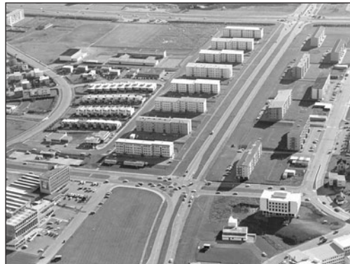
This neighbourhood has been used in an American textbook as an example of bad planning.
