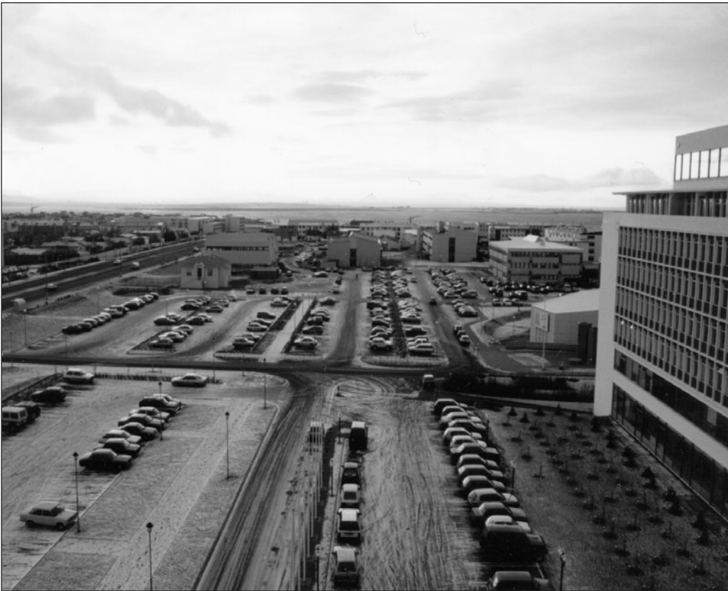
The centre of the university lies between Sudurgata street and Hotel Saga (to the right in the picture). This area, however, mainly contains cars and the buildings are at the edge. It should be vice versa.
