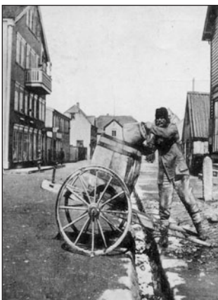
Water mains replaced delivery and pumps.
