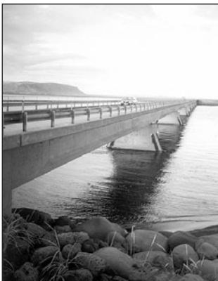
First evaluation of regional impact of a bridge was on Óseyrarbrú.
