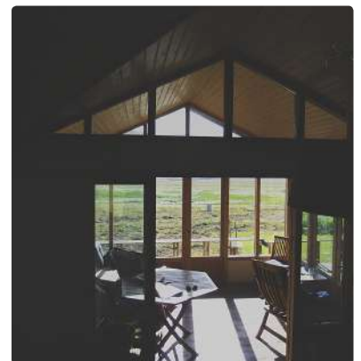
Windows under roof in hut and house
