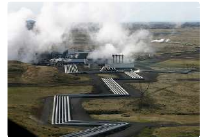
Steam can be transported long distances, but hot water even further
