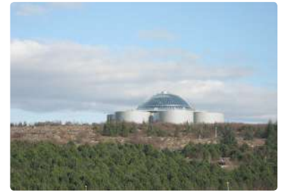
The tanks on Öskjuhlid held hot water as the flow to Reykjavik was gravity fed
