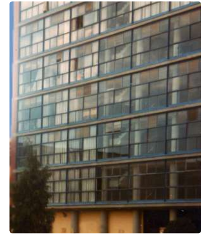
Mexico University a la Corbu. Sun kept out with paper and column area closed
