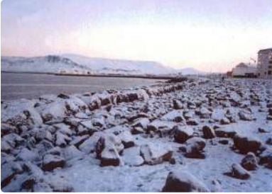
I have warned that the new landfills and breakwaters, are not high enough
