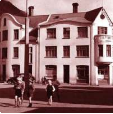
The Centre of Isafjördur is an example of pleasant town planning
